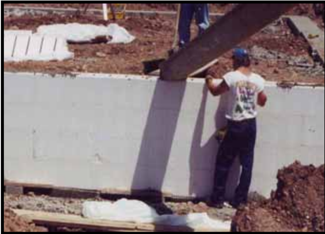
Four Foot Wall without Bracing
