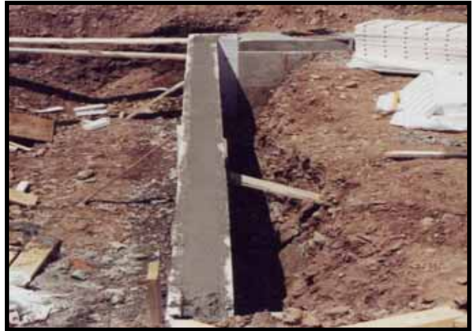
Four Foot Wall without Bracing
