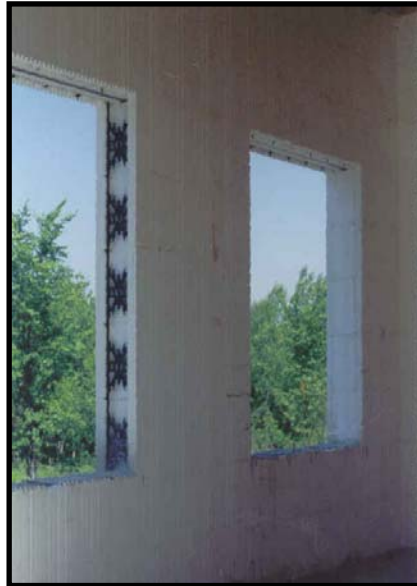
IF OVERSPAN, PLACE SPACER/WEB IN RSO AND REMOVE AFTER CONCRETE PLACEMENT
